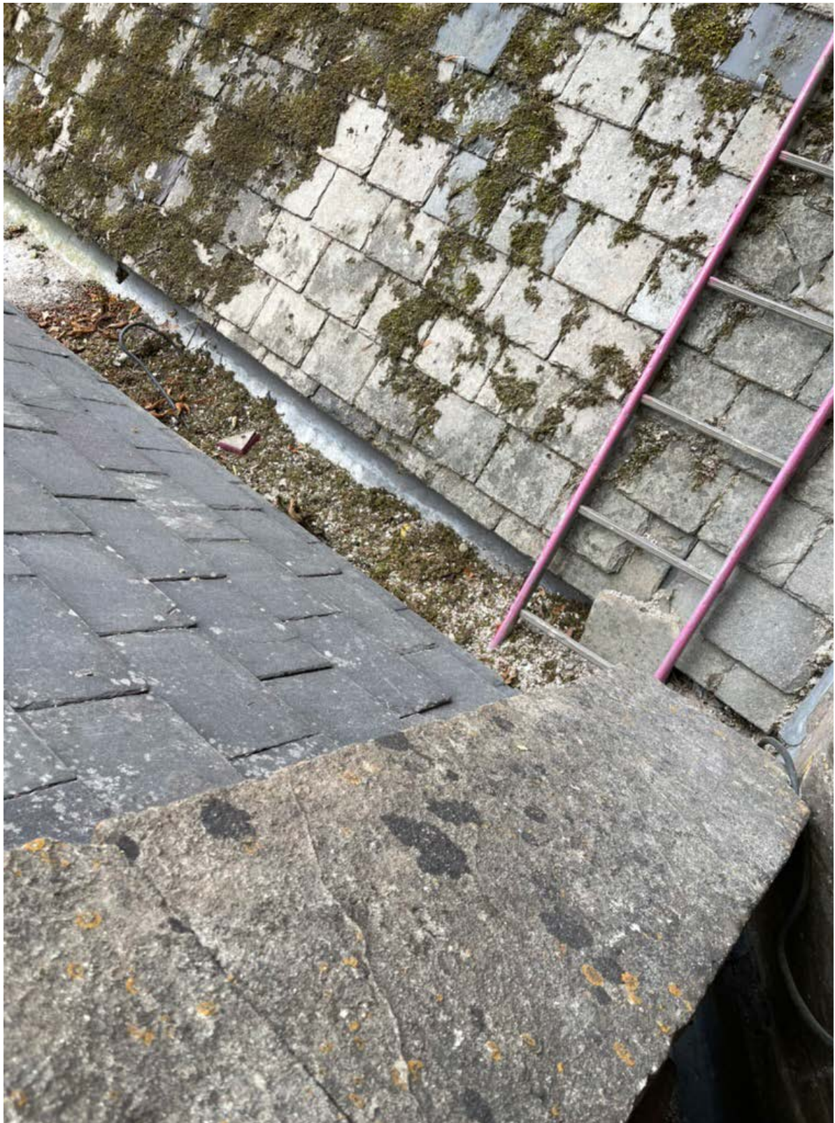
Image 2: Scaffolding ladders have been left on the roof. Small number of slates to be repaired to this area, and to the wider roof (where access permits). Large amount of build-up of moss in the lead box gutters, this has formed a blanket towards the west discharge point. The lead is to be inspected once the materials have been removed.
