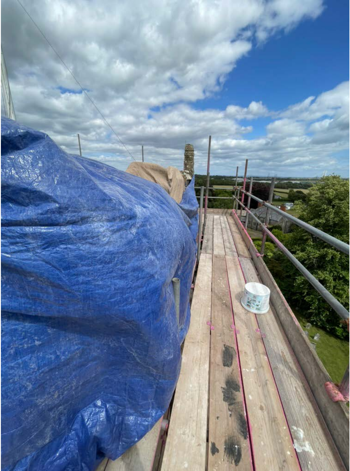
Image 5: Protection with hessian and tarpaulin to the south wall of the parapet. Lime is wetted during this stage to ensure it doesn't set too quickly.
