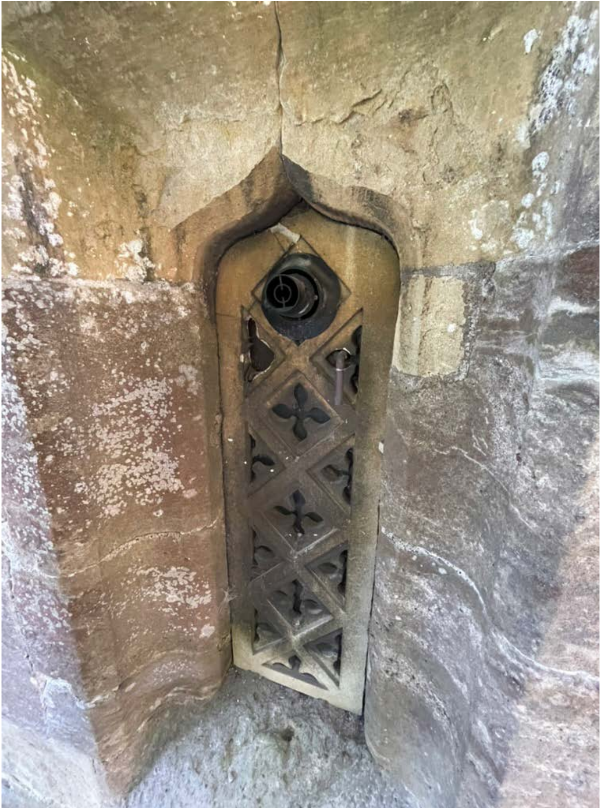
Image 6: Exhaust from the north elevation of the ringing chamber panel. Ideally would be extended.
