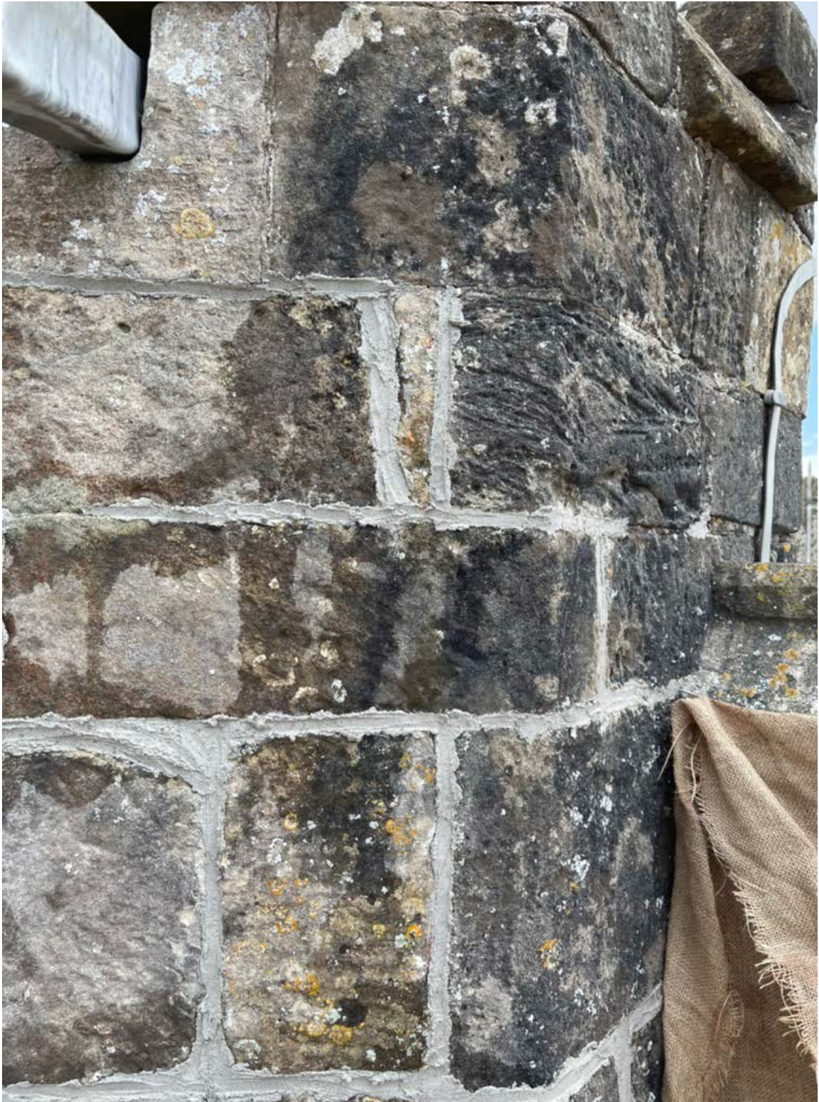
Image 3: The process of lime mortar repointing requires the lime to be tended and is not a quick process and is influenced by the weather conditions. The image above provides an example of lime most recently applied within the joint. Once this is ready and 'leather-hard' it will be knocked-back/tamped with a churn brush to expose the aggregate. Please note, this is not the final finish!
